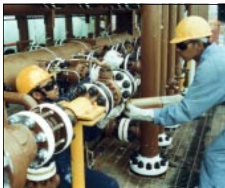
Installation of FlangeShield
