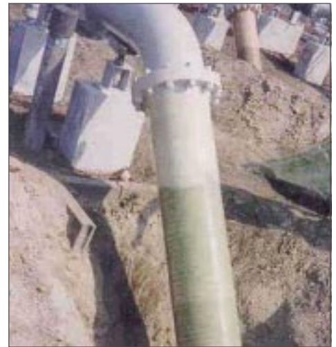
Pipeline protected with Fibaroll
